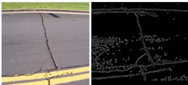
(a) (b) Figure 6: (a) original image. (b) Canny edge detected image
