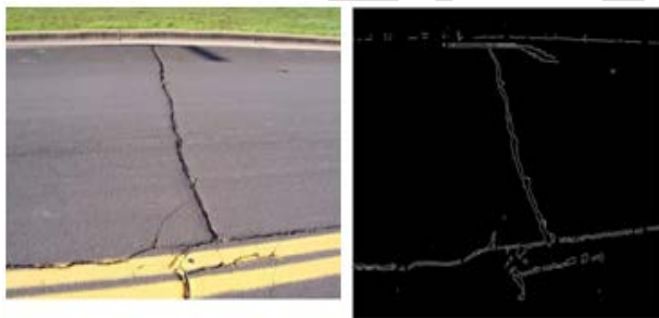
(a) (b) Figure 7: (a) original image. (b) sobel edge detected image
